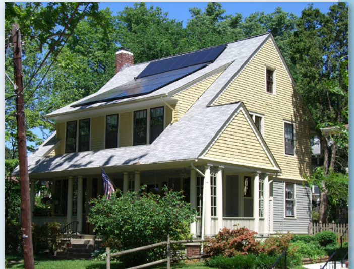
A 6-kW PV system provides 85 percent of this Washington, D.C. home's electricity. Courtesy: Standard Solar
