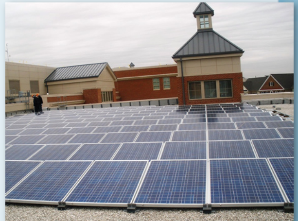
Just outside Washington, D.C., Lakelands Park Middle School in Montgomery County hosts a 111-kW rooftop PV system, deployed under a solar PPA with SunEdison. Courtesy: SunEdison
