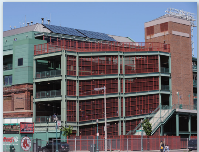
Solar water heating system installed by groSolar on Fenway Park provides one third of the stadium's hot water.
