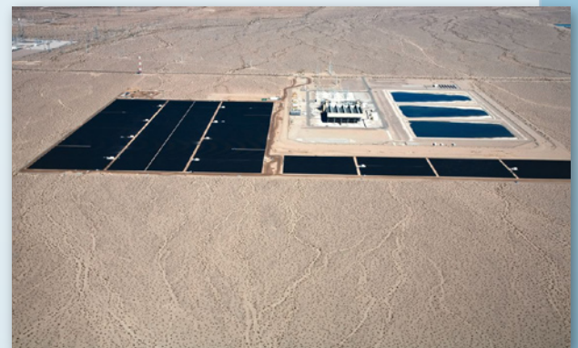
El Dorado 10-MW AC PV plant near Boulder City, Nev.
