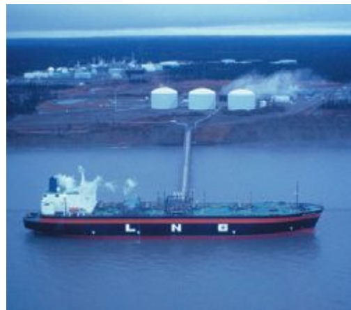
An LNG plant at Kenai, Alaska, US. The market share of natural gas is expected to increase from 19% in 2002 to nearly 30% in 2030, much of this increase due to the rising demand from India and China (ConocoPhillips)
